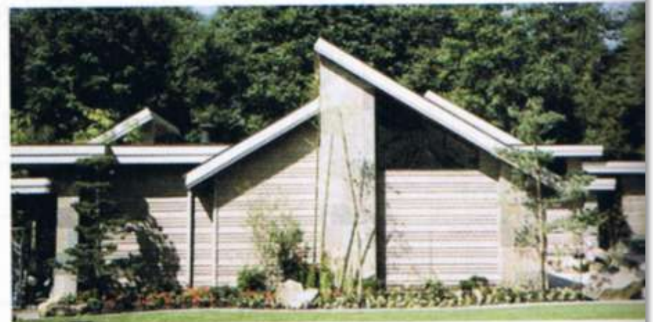
FIGURE 20.10 ■ Many contemporary homes combine flat and shed roofs to create a pleasing design. Courtesy LeRoy Cook.
