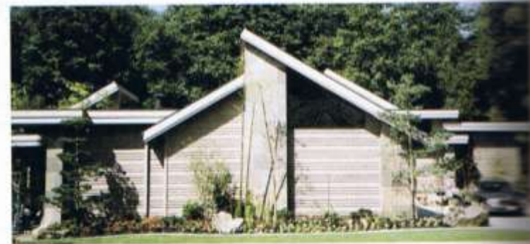
FIGURE 20.10 ■ Many contemporary homes combine flat and shed roofs to create a pleasing design. Courtesy LeRoy Cook.
